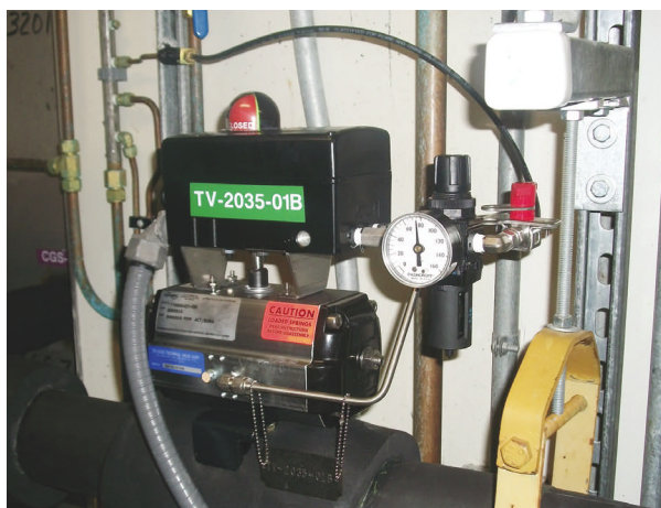
Knew Buffer Prep Tank Cold Glycol Temperature Control Valve: After
