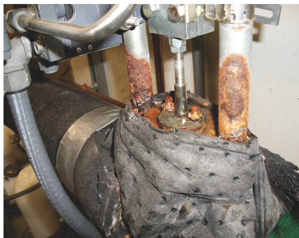
Close-up of a Typical Buffer Tank Glycol Temperature Control Valve: Before
