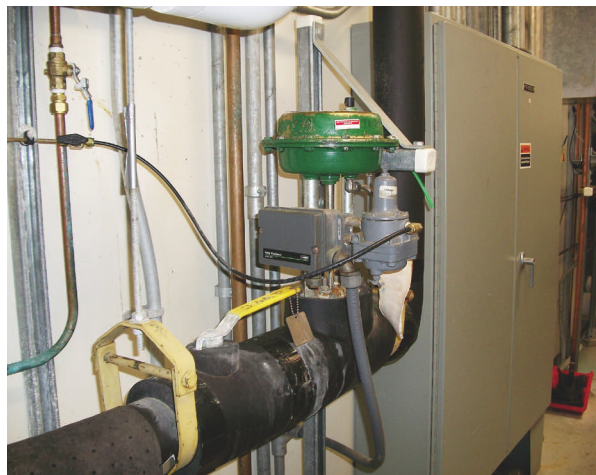
Original Buffer Prep Tank Cold Glycol Temperature Control Valve: Before
