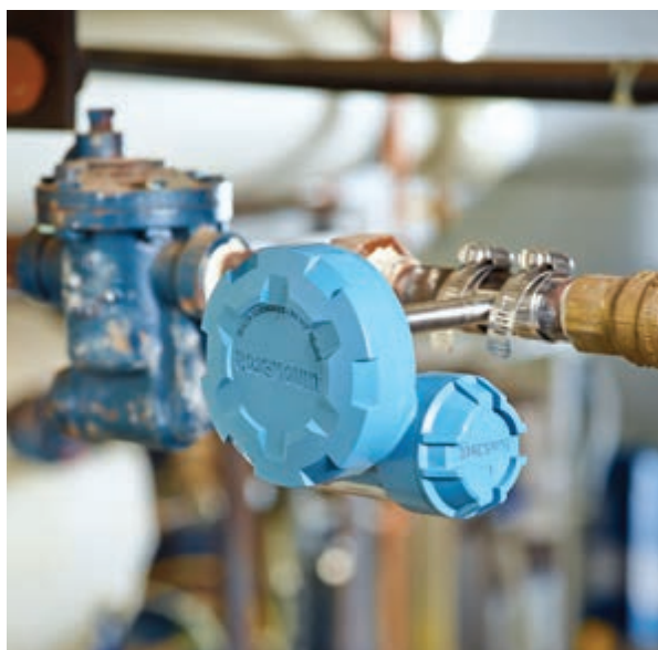
Figure 1: Acoustic monitors can work with many different types of steam trap configurations.
