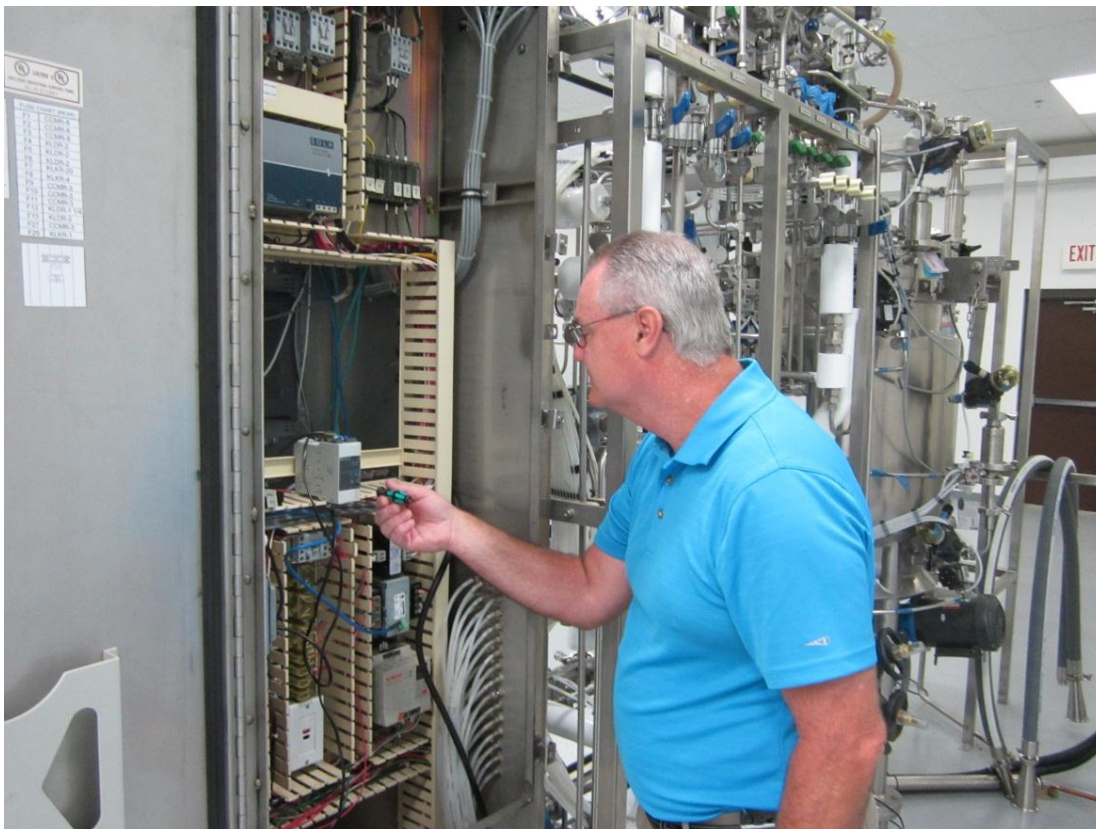
Figure 6: A partial proof test can be initiated by pushing a button on the Nivotester receiver or on the level switch.
