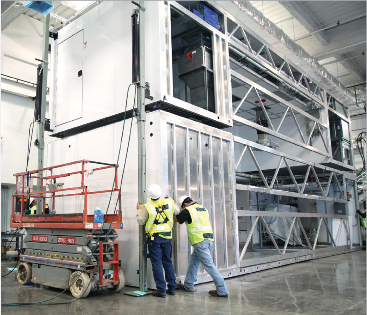
Assembly of the megaPOD; top section, left, lifted and bottom section, left, being moved into place (Courtesy of G-CON Manufacturing Inc.)
