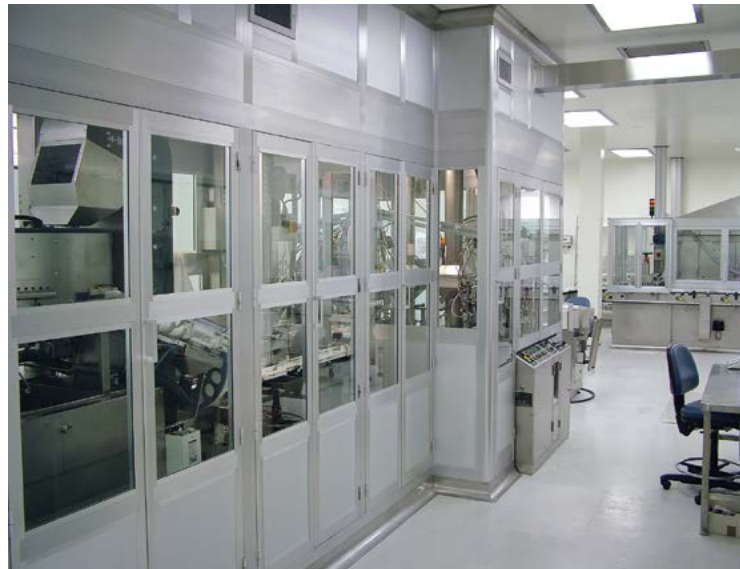
Part of Catalent’s Pressurized Metered Dose Inhaler (pMDI) filling suite at RTP, North Carolina.
